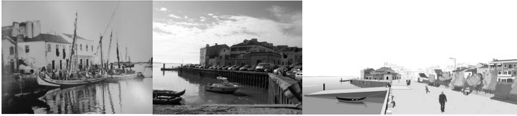
Figure 4. The old river port (1920’ photo; existing; visual simulation of design renewal)
