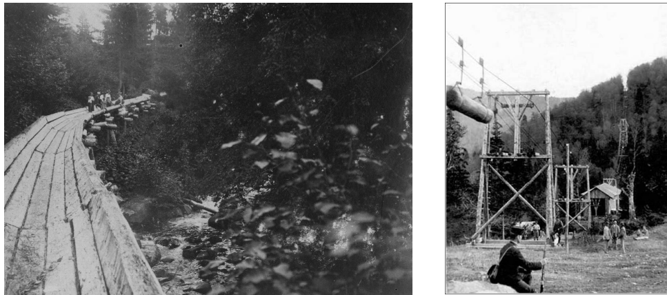
Figure 1. Skid-row and trunk lift, belonging to the Mikes Estate (Source: The Archives of Mikes-Chowdhury Family, Zabola )
