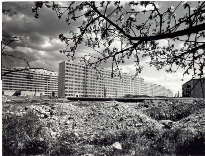
Figure 1. Housing estate under construction in the 70-s
