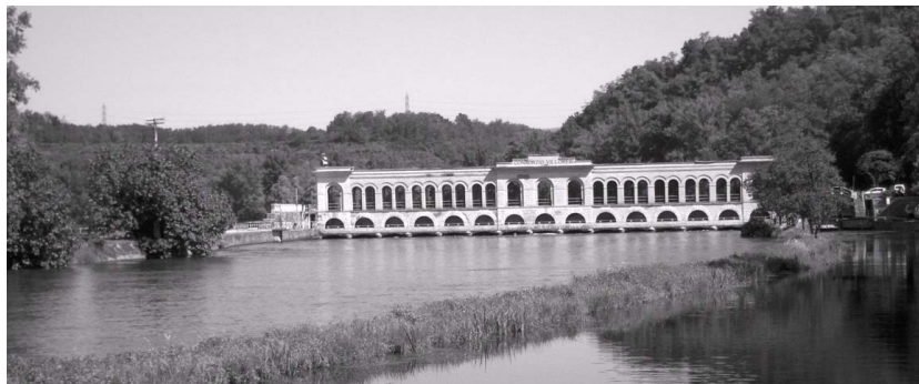
Figure 1. Panperduto Dam on Ticino River (C. Pisoni picture)
