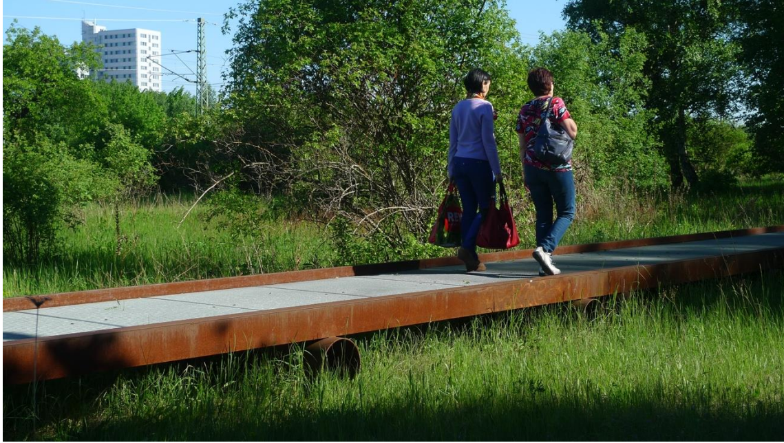
Figure 7. Raised steel walkway provides elegant passage across fragile and rare spontaneous grassland habitat.
