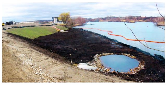
During construction, the bank was relocated by 26' and extensive care was taken to clean toxic soils and provide the foundation for a renewed ecosystem.
