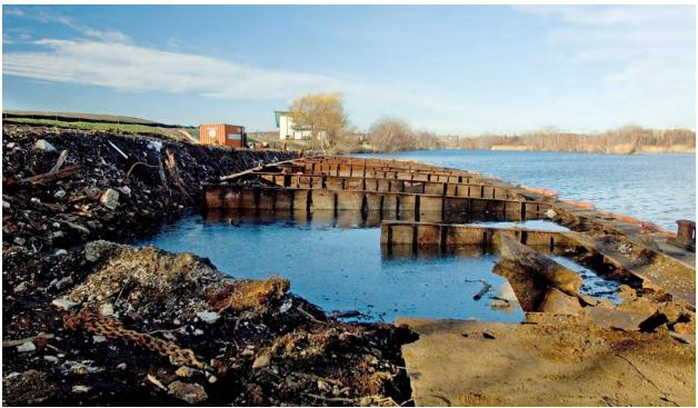
This view shows the site after removal of derelict buildings but prior to removal of the 100-ton, 40' x 270' sunken, and garbage filled barge. Landfill soils were typical of the entire riverbank. Over 17,000 tires were recycled. The nearly completed Tufts University Boathouse is in the center of the photo.
