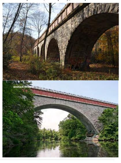
carry water from the Sudbury River to Boston. Constructed in 1876, the stone and brick bridge is 475 feet long and 19 feet wide, with seven stone arches.
