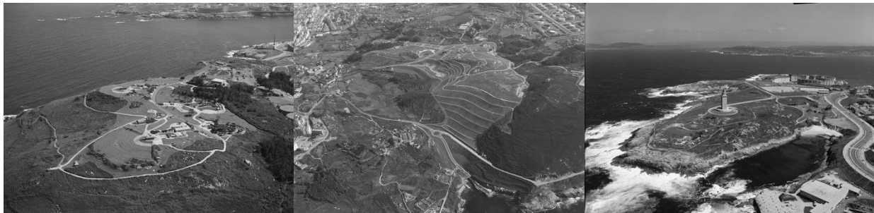
Figure 3. San Pedro Park (old military battery), Bens Park (old municipal garbage dump), and surrounding area of the Torre de Hércules (World Heritage).
