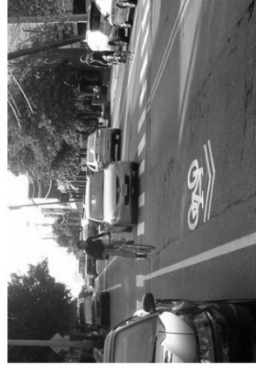
30. Shared lane markings provide guidance on roadways that are not wide enough for bike lanes.
