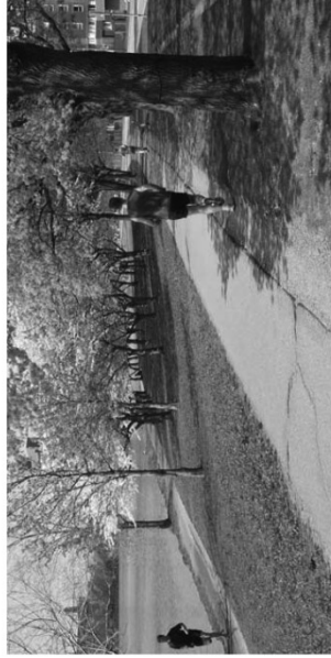
User-created "goat tracks" occur when users feel that the path surface provided is too narrow, too hard or both. Here, three informal paths have been created.
