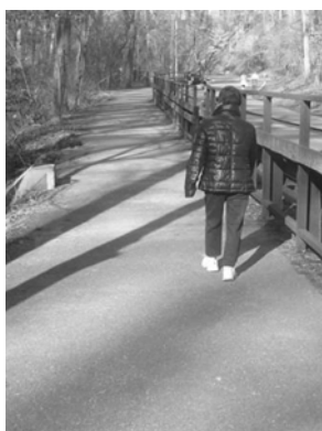
Figure 3. Example 1 of Co-Aligned Trail and Roadway Condition
