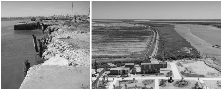
Figure 3. Tagus Linear Park; before (left) and after construction (right)
