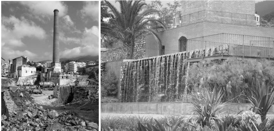
Figure 1. Santa Luzia Gardens; before (left) and after construction (right)
