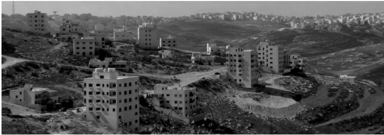
Figure 5. Area 3, photo by the authors
