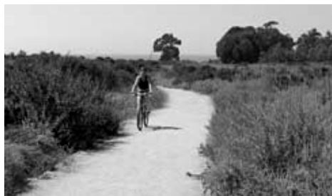
Fig. 17 Carpinteria Bluffs Coastal Vista Trail, Made of Stabilized Decomposed Granite
