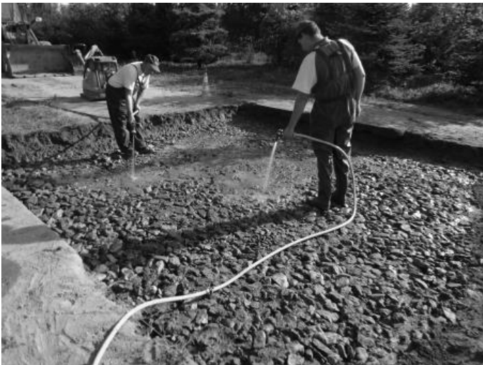
Figure 1. Filling the vegetation layer with substrate using the water
