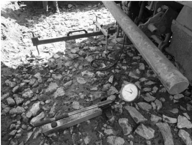
Figure 2. Bearing capacity examination of coarse aggregate layer
