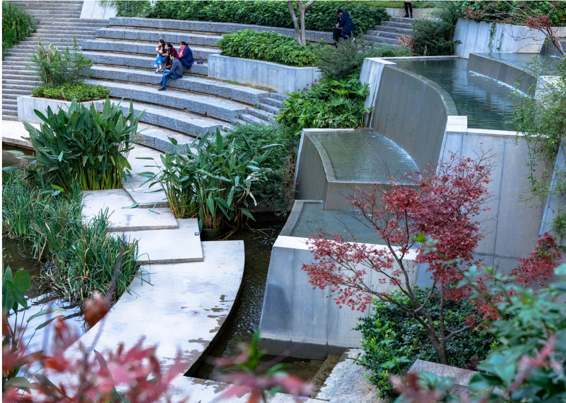
Fig. 3: The grading, elevation, levee, and planting were designed to withstand the storms and flooding common to the area. The amphitheatre and planting can endure full submersion in the event of a flood.
