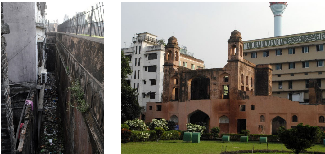
Figure 5. Encroachment along the South wall and Gate (Source: author)
