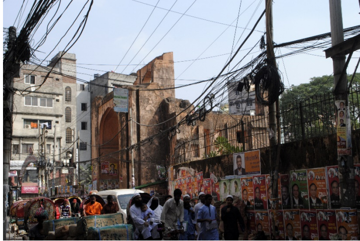
Figure 6. Outer Wall Covered with posters (Source: author)
