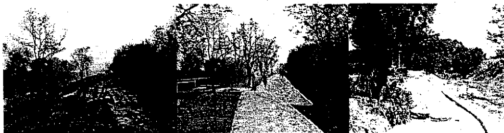
The Greenway of Alpiarça Royal Canal: existing condition: visual simulation: construction works
