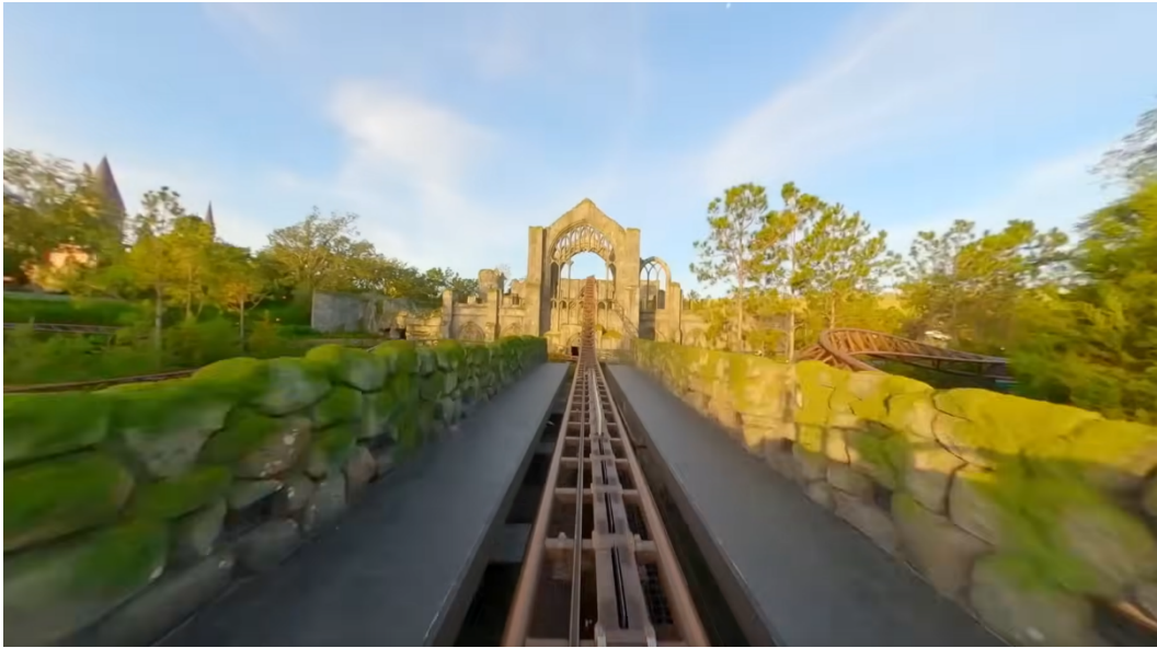
Figure 4 – View down LSM launch track, HMA
