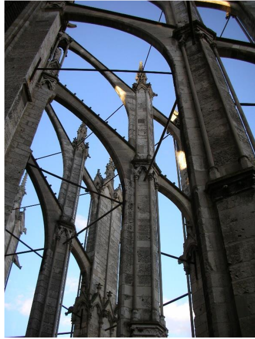
Figure 1: Beauvais Cathedral buttresses and reinforcement, Accessed May 3, 2021, https://phys.org/news/2014-12-gothic-cathedrals-blend-iron-stone.html
