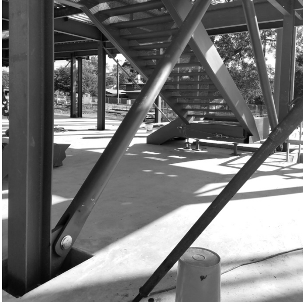
Fig. 5. Bracing detail during construction (by Kevin Crumley)
