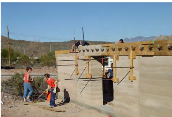
Figure 5: Third rammed earth project in construction; with pipe clamps supporting the continuous formwork for a bond beam.
