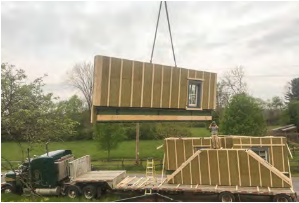
Figure 6: GoHome Panelization House Assembly Process
