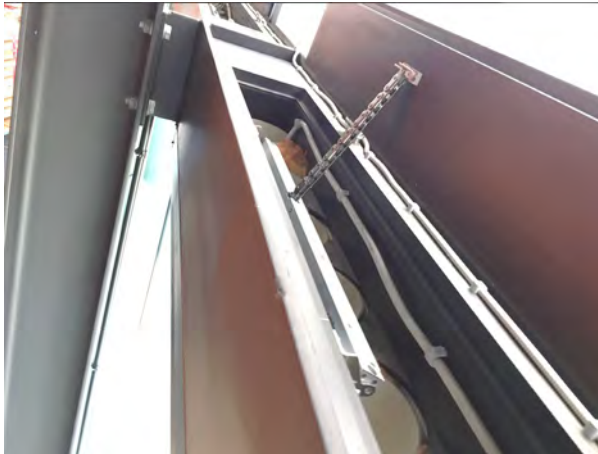
Fig. 7. The bay-width-sized ventilation flap in open position with one of its two 24V motor.
