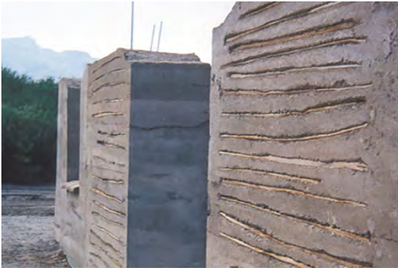
Figure 4: Gila River dwelling with saguaro ribs embedded in entry wall.
