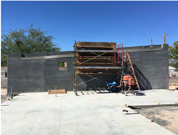
Figure 8: Scoria walls with incremental bond beam.
