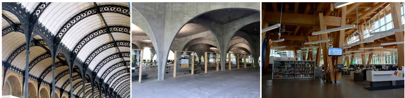
Fig 1: Ste. Genevieve Library, Paris (iron), TAMA Art Library, Tokyo (reinforced concrete); Scarborough Library, Toronto (timber). As can easily be seen by the above three images of libraries, materiality plays strongly into form, feeling and detailing in spite of programmatic similarities. A high level understanding of materiality was required of the architect. Photos by author.
