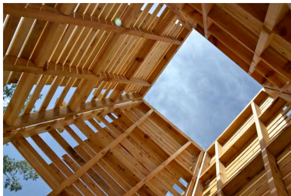
Fig. 2: Displacement Analysis for the Kilim project and a view from inside one of the two observation towers
