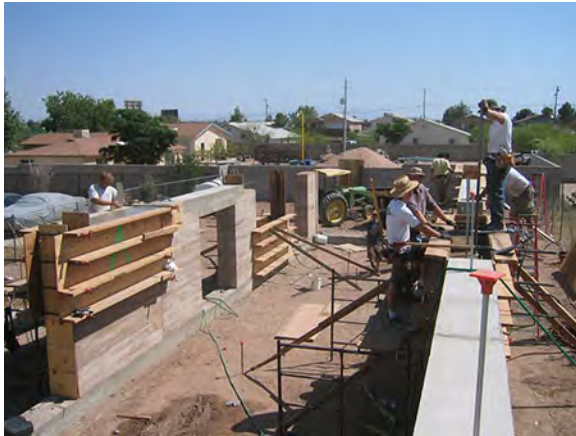
Figure 6: Incremental bond beam construction in Project 4.
