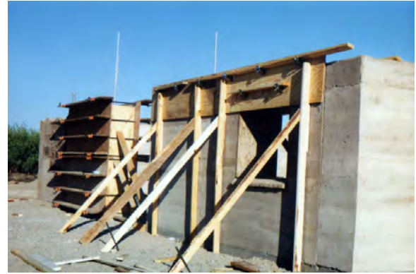
Figure 3: Second rammed earth project in construction, showing end boards and movable forms.
