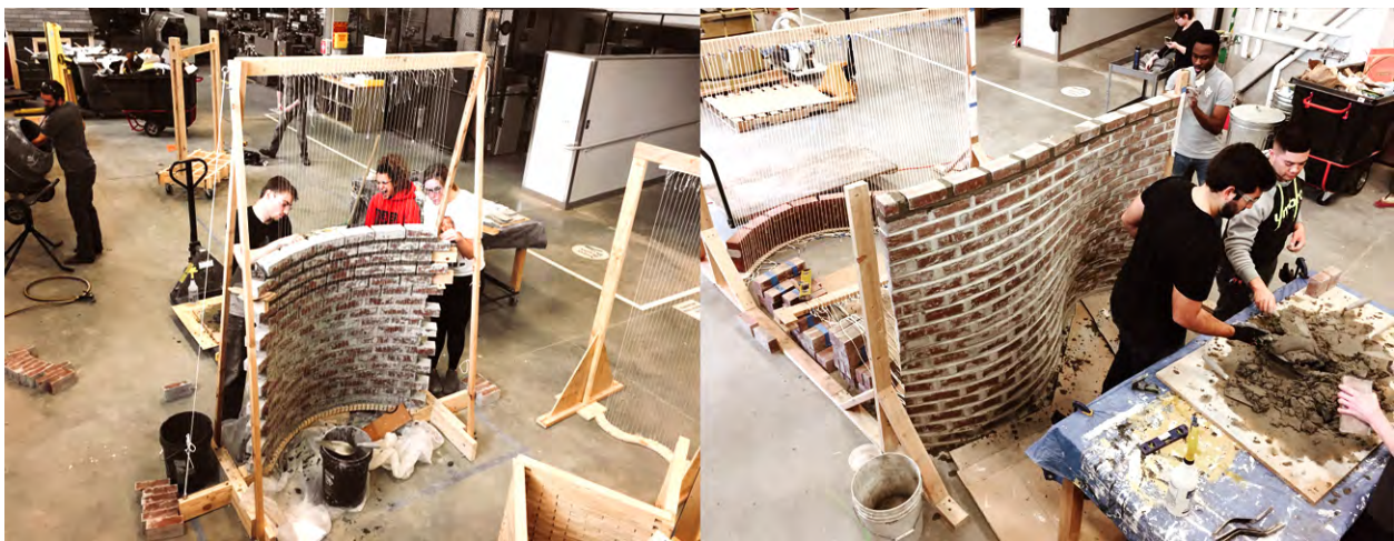
Fig. 4. Dieste Building Shop - Ruled Surface Wall Construction
