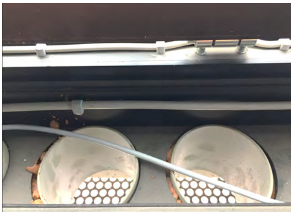
Fig. 8. View from above of two air inlets lined with short PVC stub. The slightly larger diameter cutout in the HEA240 is visible as is some sprayed-in foam insulation filling the lower cavity beneath the shape's web. The perforated closure angle is visible, but the insect screen resting directly on it is washed out in this photo by the author.
