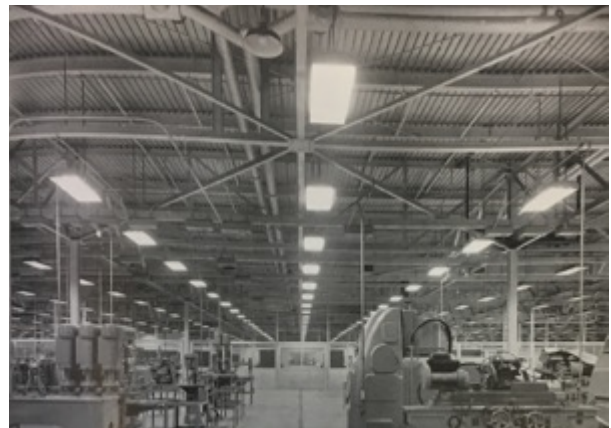
Fig. 2. Austin Company's design for the Allison division of General Motors was among the first to use fluorescent fixtures throughout. Architectural Record, February, 1940. 91.
