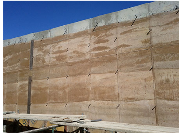
Figure 7: Rammed earth wall of Project 5; this wall constructed with industrial forms.
