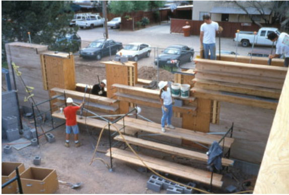
Figure 2: First rammed earth project in construction, showing VDBs and movable forms.
