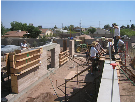
Figure 6: Incremental bond beam construction in Project 4.
