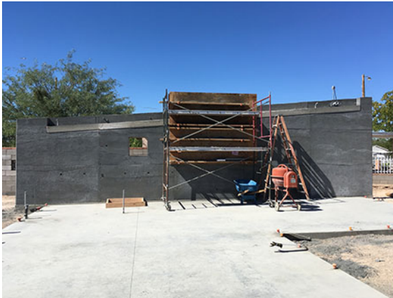
Figure 8: Scoria walls with incremental bond beam.
