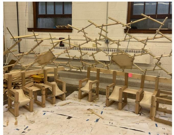
Fig. 9. Team 2 used augmented reality to project the 3D model of the reciprocal frame and build the prototype
