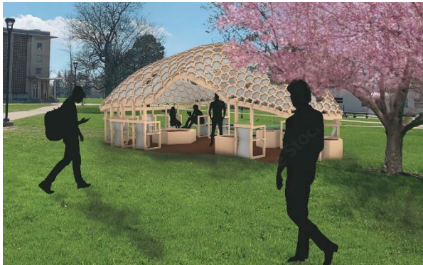
Fig. 8. The reciprocal frame developed by Team 2 as their second prototype. Source: Emily Connor Vollo, McCormick, and Jacob Maciejewski
