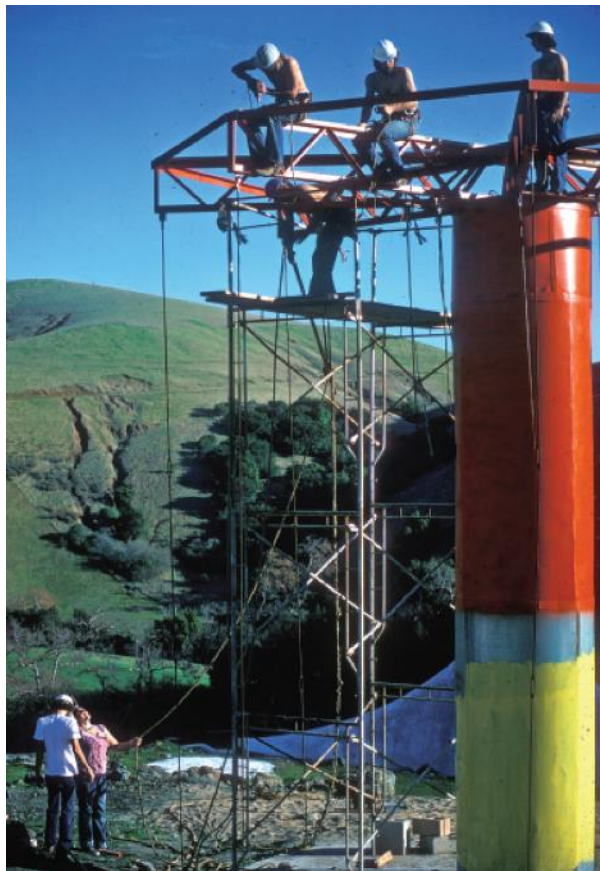
Fig. 2. Photograph of the Fluid Column during installation of the roof truss system, 1974. Courtesy Dr. Jens Pohl.
