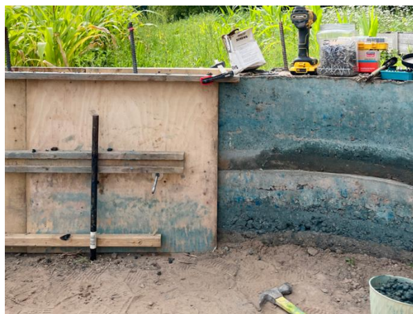
Image 3. Formwork in the rammed-earth construction process.
