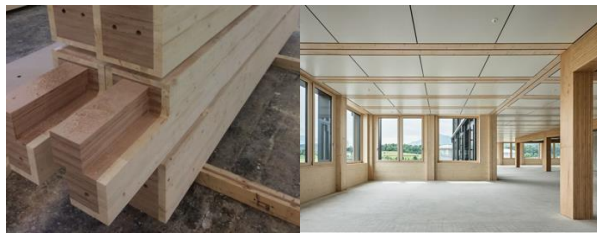
Fig. 3, (left) Pollmeier BauBuche Beech LVL column with spruce. Photo Credit: HESS Timber
