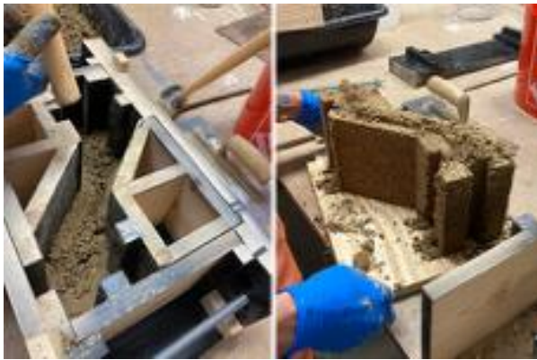
Fig. 12. Zig Zag shape earth block fabrication.
