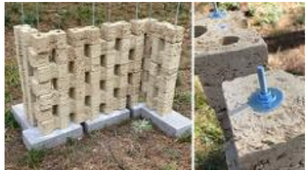
Fig. 6. Wall construction – all-thread rod and fasteners.
