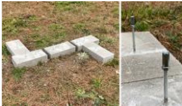
Fig. 5. Wall construction – foundation and anchor bolts.
