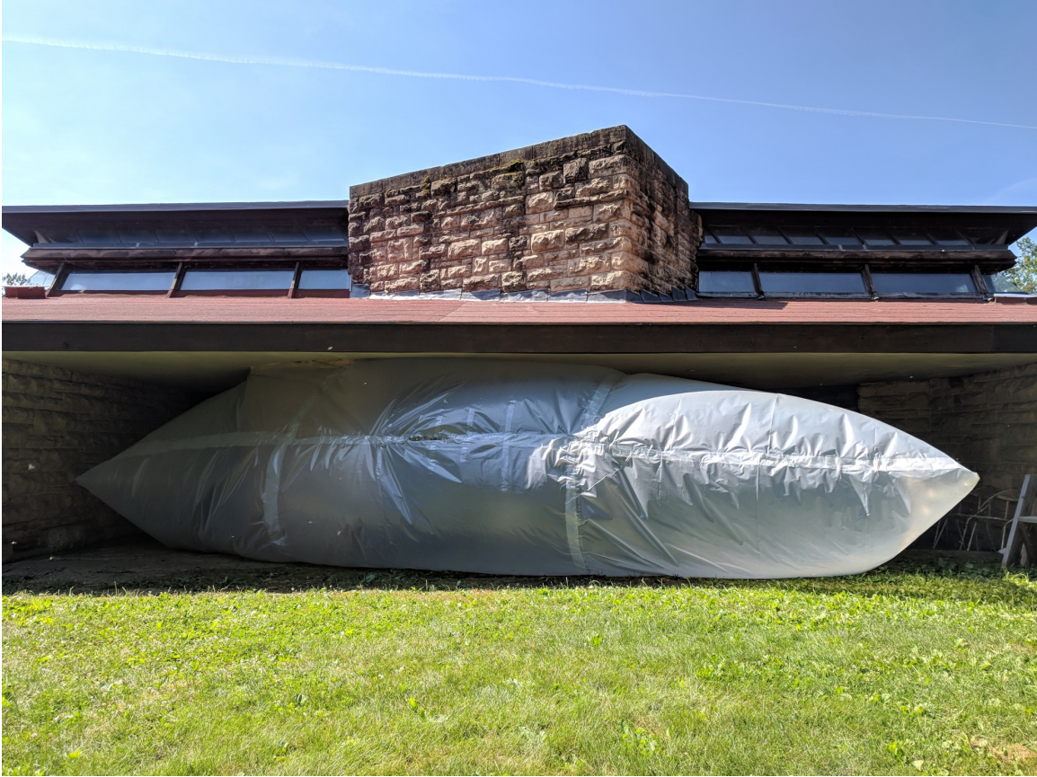
Figure 1: Inflatable wedged under the north porch and encompassing the hearth of the Hillside Home School (II) designed by Frank Lloyd Wright at the Taliesin estate in Spring Green, Wisconsin. Source: (Author 2018)
