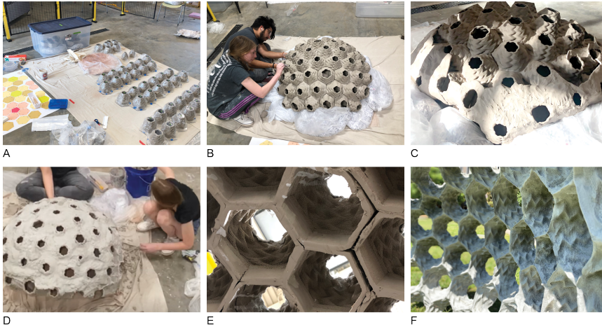
Figure 8: Image A shows the 52 units. The plastic keeps them from drying further as they are assembled. A diagram denoting the assembly logic can be seen in Image A. Image B shows the students constructing the formwork, and Image C shows the additional clay added to prevent leaking. Image D shows students removing the clay formwork. The clay is beginning to dry and fall off in image E. The final cast is displayed in image F. Work by Haley Arthur Eisenmann. (Haley Arthur Eisenmann 2022)
