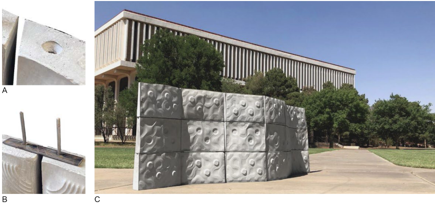
Figure 6: Image A shows the hole left within the cast for the welded connection (B). This welded component holds the tiles together. Photo C shows the final wall—work by Adrian Reyna. Source: (Adrian Reyna 2022)
