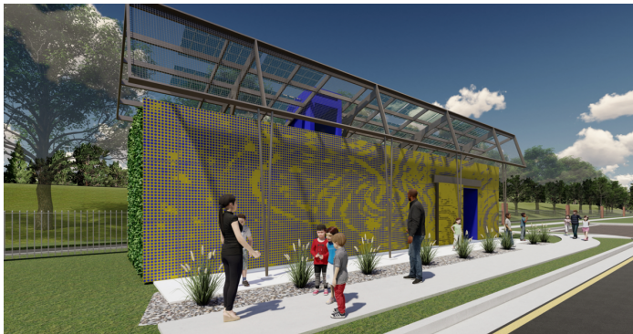
Figure 12 Rendered View: North Elevation with Perforated Rain Screen + Vertical Vegetal Wall (Michael Carroll 2022)
