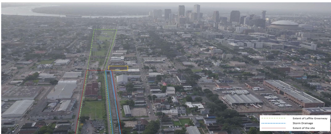
Figure 7: Drone photo of the site. Source: (Authors 2022)
