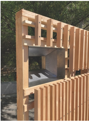
Figure 18: Frame-Opening Final Assembly with Expressed Fasteners. Source: (Author 2022)
