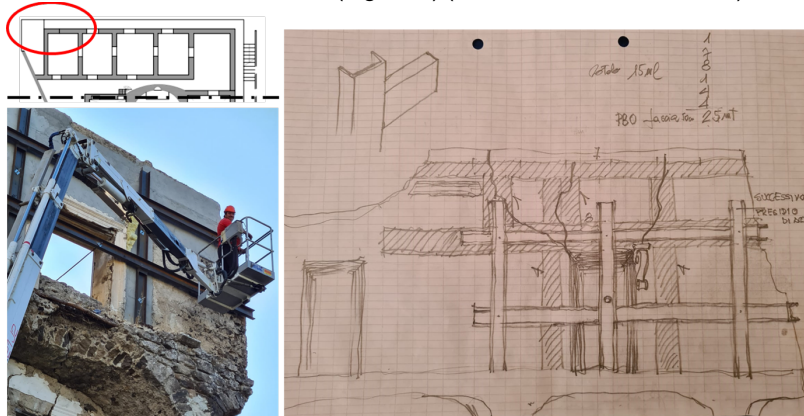
Figure 7: Securing unstable Eastern masonry edge (Source: Authors 2022)
