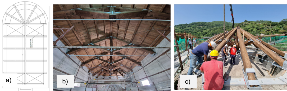
Figure 5: Timber roof structure. a) Roof scheme b) Central nave rood c) "umbrella-knot" (Source: Authors 2022)
