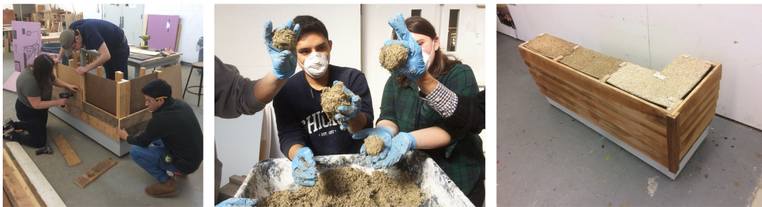
Figure 6: Mockup wall construction. Source: (Author 2019)
