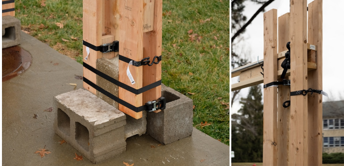
Figure 3: Non-intrusive assembly connections using ratchet straps. (Author 2022)
