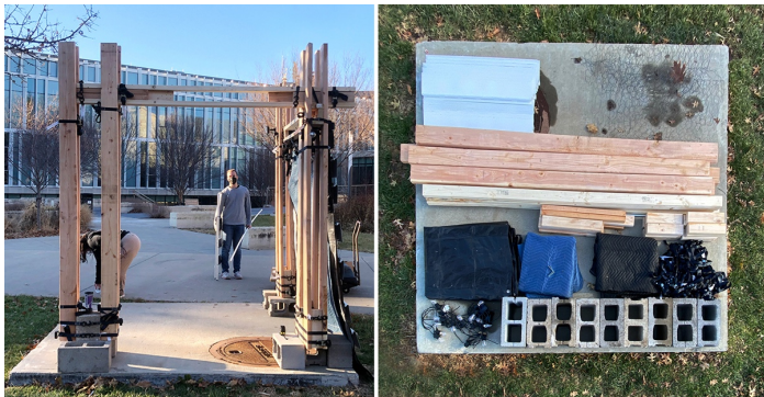
Figure 4: The assembled wall structure and their components after disassembly. (Author 2022)
