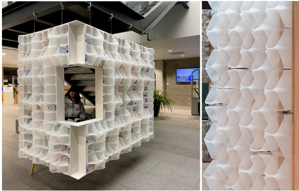
Figure 6: Reused plastic wall installation suspended under a library staircase. (Author 2022)
