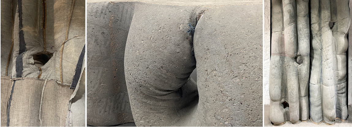
Figure 8: Precast concrete panel from fabric waste formwork. (Author 2022)
