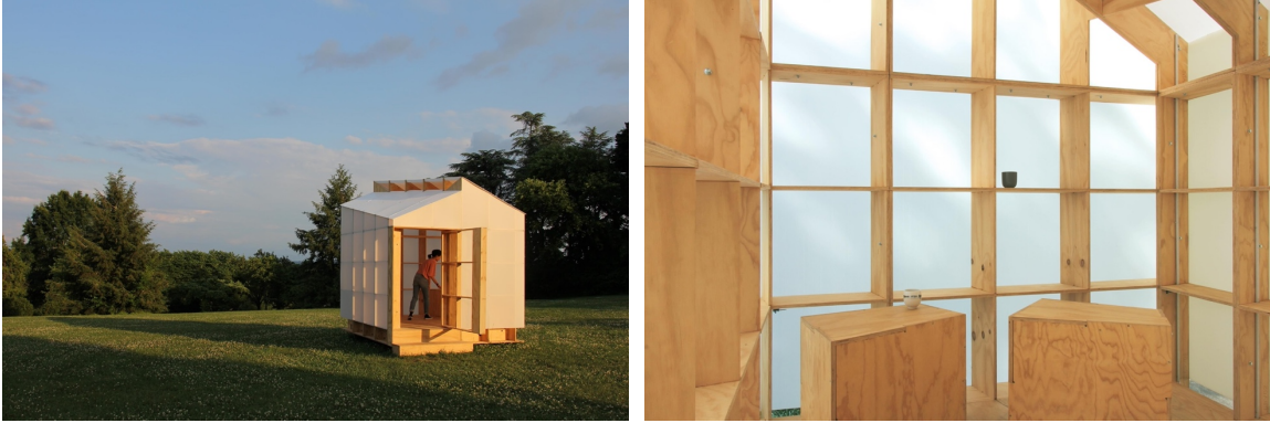
Figure 7: Occupants can modulate the structure's thermal performance through operable doors and openings. Source: Authors; and the installation's translucent and lightweight skin allows occupants to engage with the environmental conditions of the site context. Source: Authors
