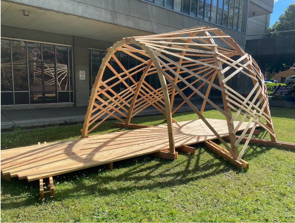
Figure 7: Final Installation. Source: (Sprague 2022)
