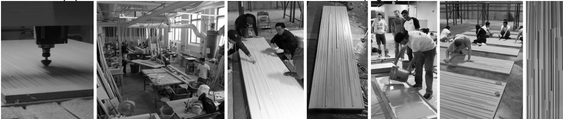
Figure 4. CRETE House . Formliners fabrication process led by students (Photographs by author).
