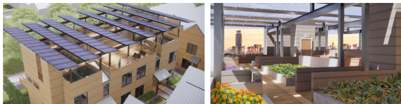
rooftop PV panels mounted on shading pergola above the Soleil flats garden roof deck.
