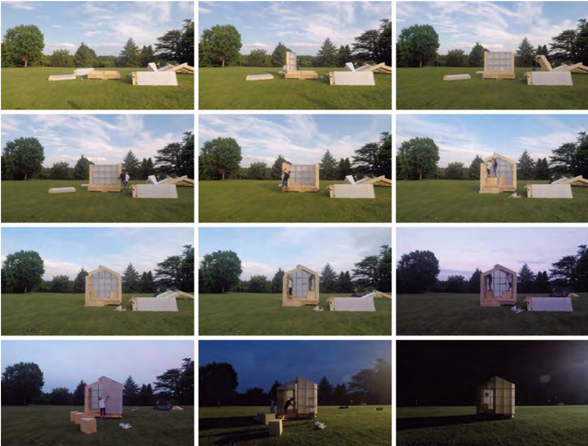
Figure 6: The integration of digital fabrication methods and construction practices enable the structure to be built in a single day. Source: Authors
