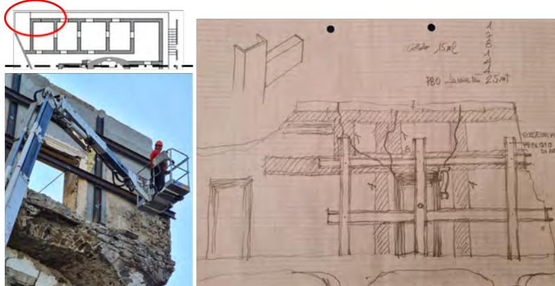
Figure 7: Securing unstable Eastern masonry edge (Source: Authors 2022)
