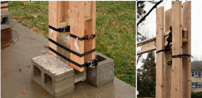
Figure 3: Non-intrusive assembly connections using ratchet straps. (Author 2022)
