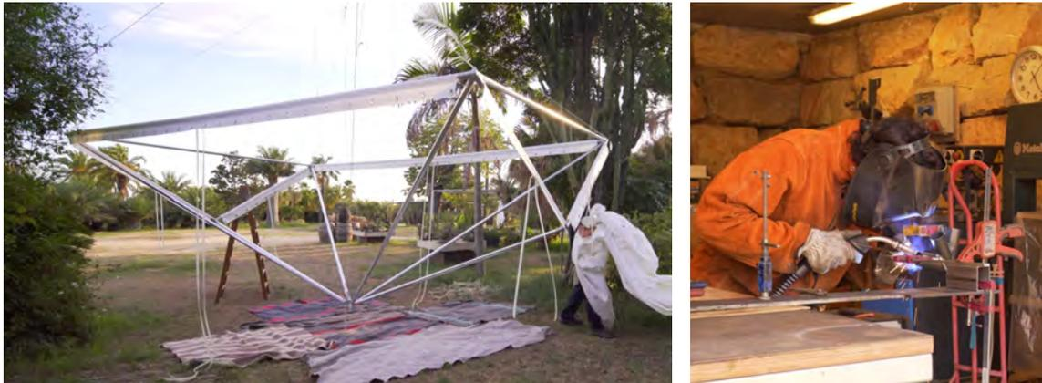
Figure 4: left: space frame mock-up, right: manual welding of steel knots. Source: (Frau Recerques Audiovisuals 2022)
