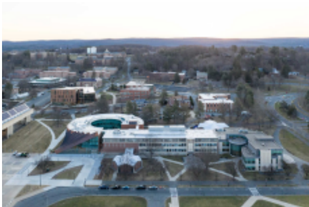
Image one: Aerial view of the old Isenberg (right) along with the new addition (left). 6
